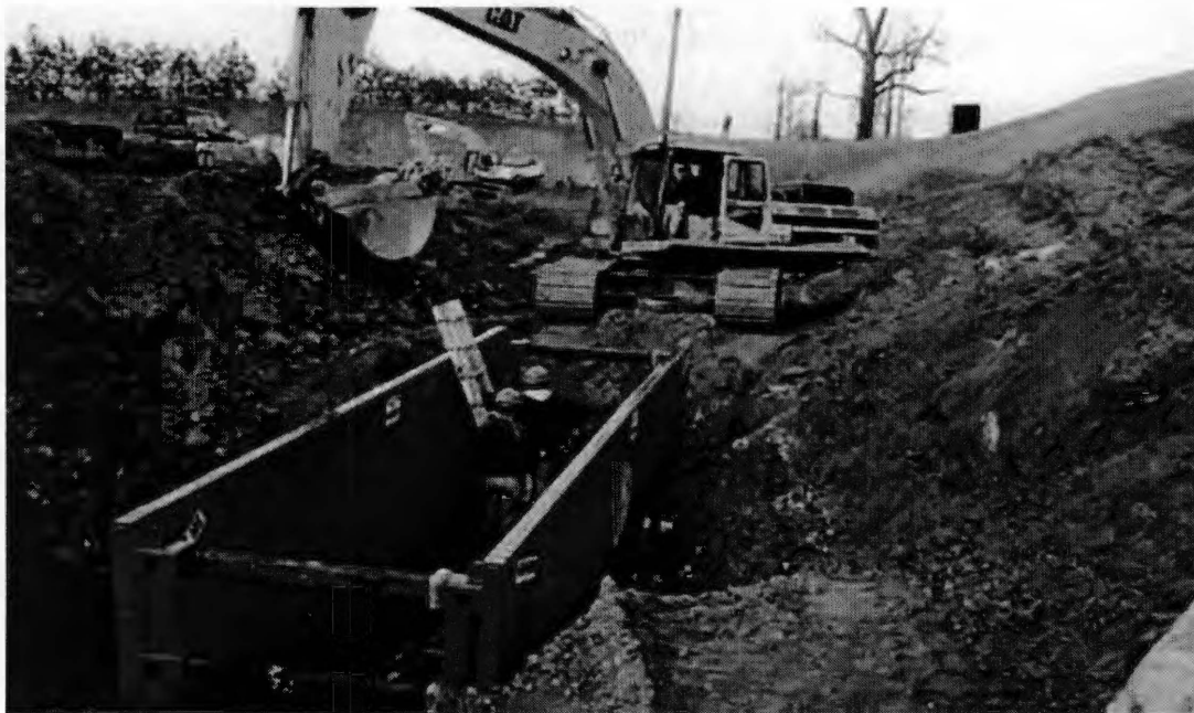
Figure 2 - Example of a Trench Box in Use
